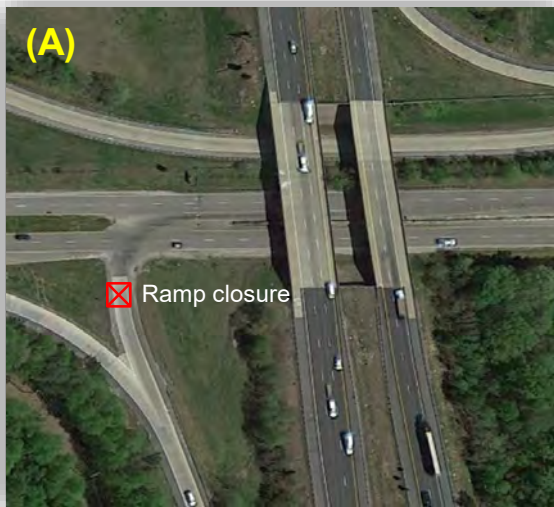
(A) A note for closing the left-turn lane on the cross road is NOT provided.
