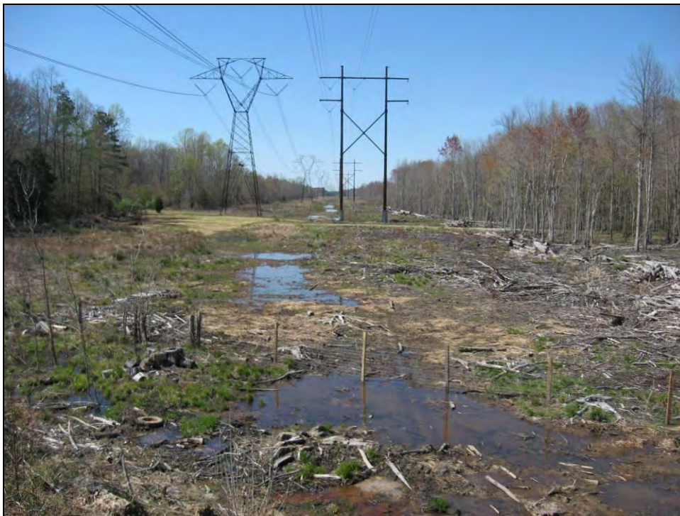
Photo 5: View of Overhead Utility Line Corridor, Facing North.
