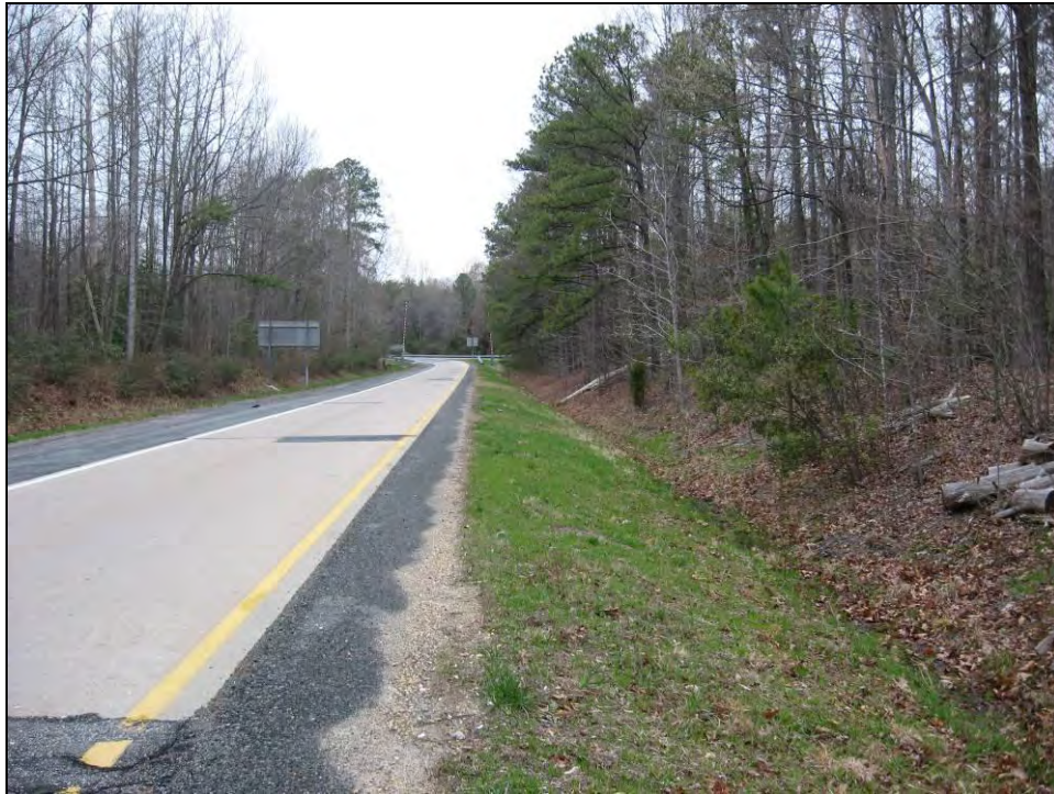
Photo 4: View of Graded Highway and the Edge of Exit Interchange 49 Ramp, Facing Southeast.
