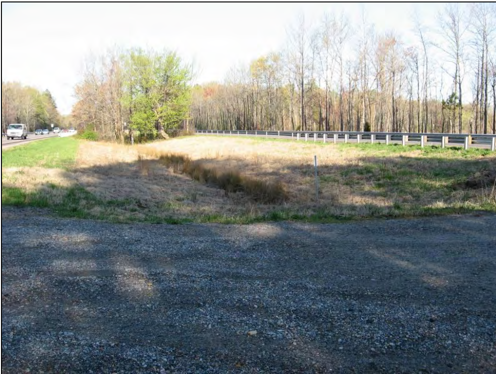
Photo 16: View of the I-64 Median and Travel Lanes, Built on Fill, Facing Southwest.
