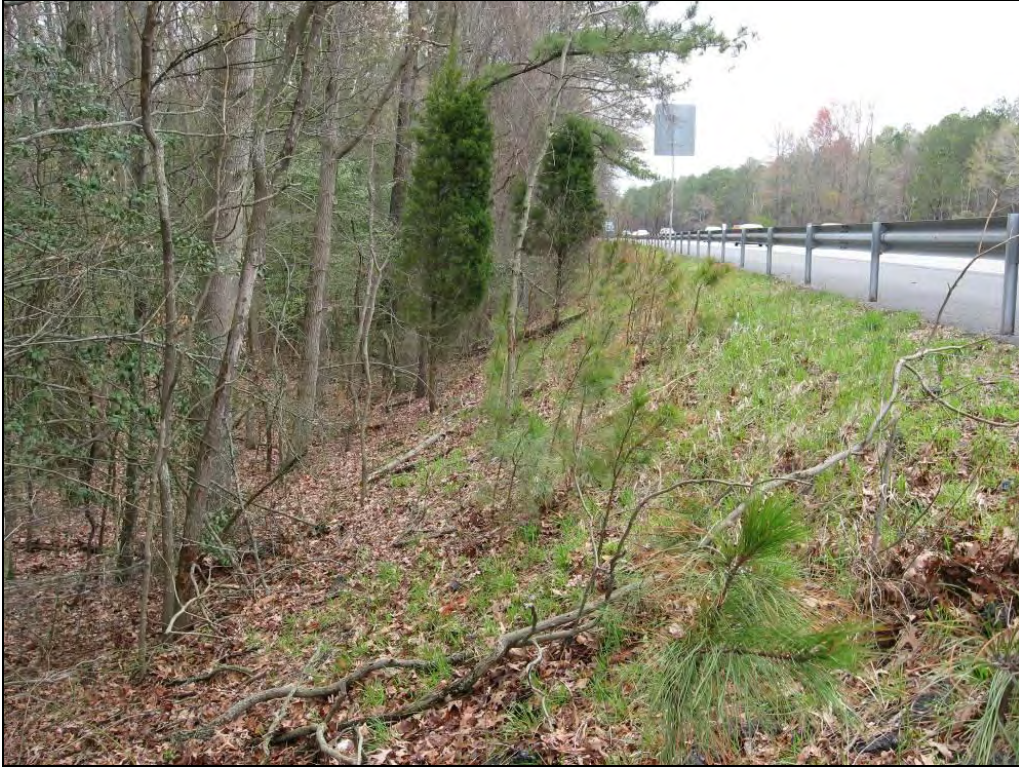
Photo 15: View of Fill Section Along the I-64 Corridor, Facing Southwest.
