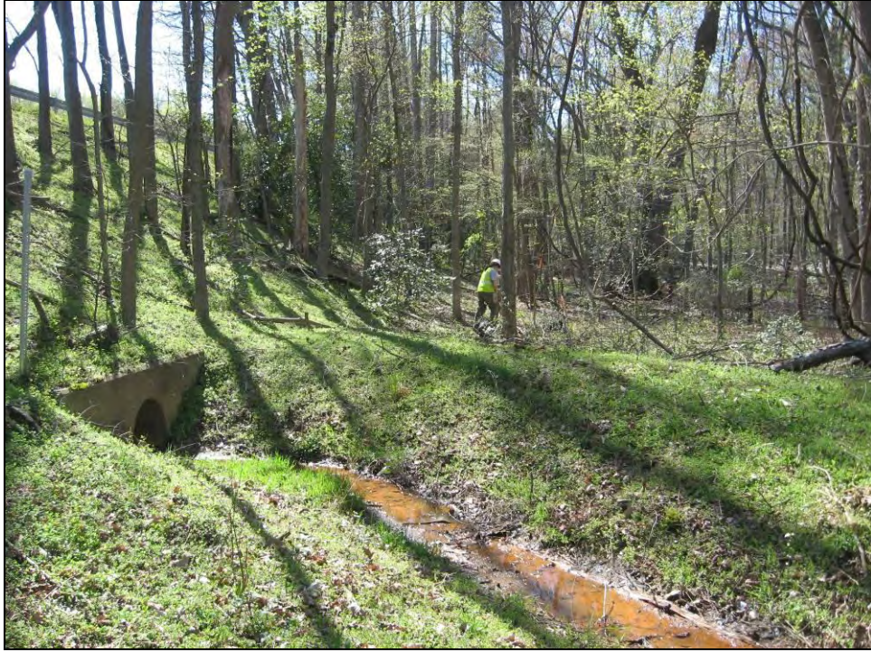
Photo 8: View of Construction Drainage within the Site Boundary, Facing Southwest.
