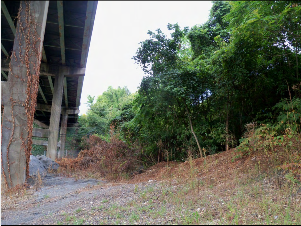
Photo 1: View South Across the Area Tested.
