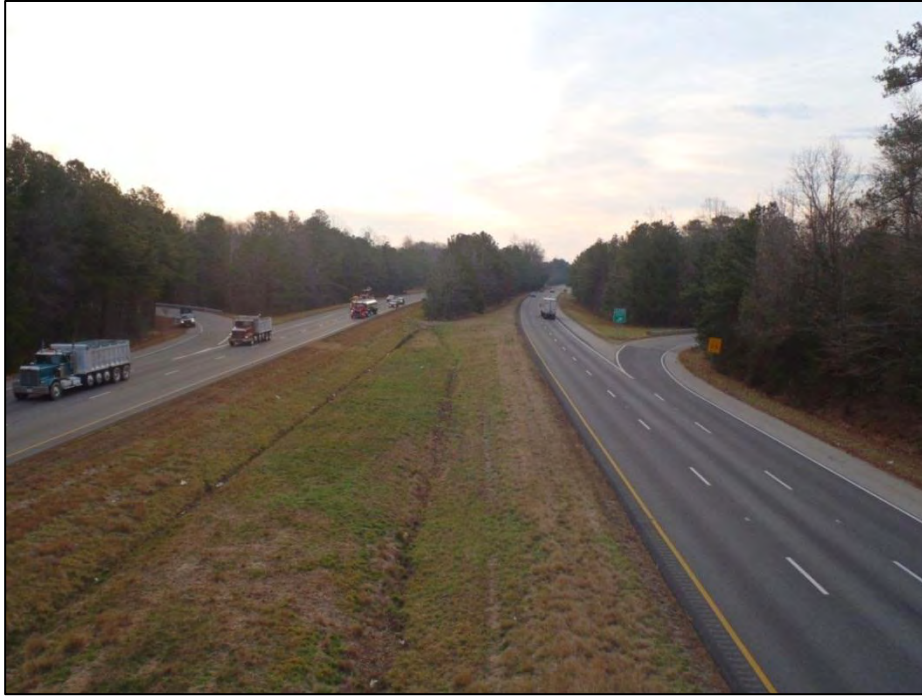
Photo 5: View East from Croaker Road Showing the Drainage Ditches in the Median.
