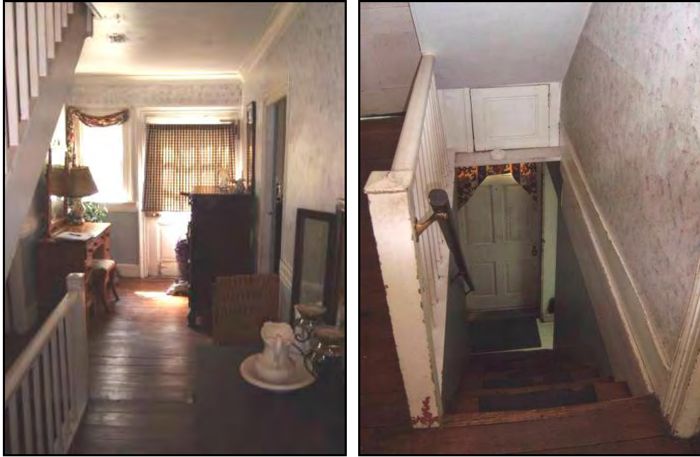
Photo [GROUP] 9: [LEFT] View Along Central Hall Towards Main Entrance on First Floor; [RIGHT] View Down Stairwell to Basement Level (Dovetail, Sep. 2011).
