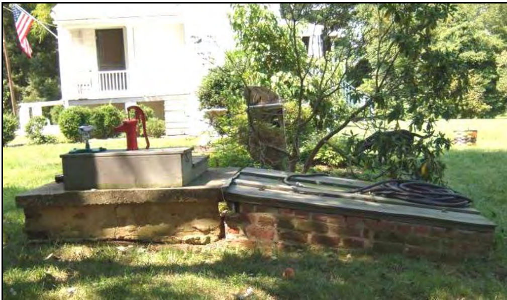
Photo 14: Overview of Brick Well and Cold Storage Cellar East of Main House, Looking West (Dovetail, Sep. 2011).
