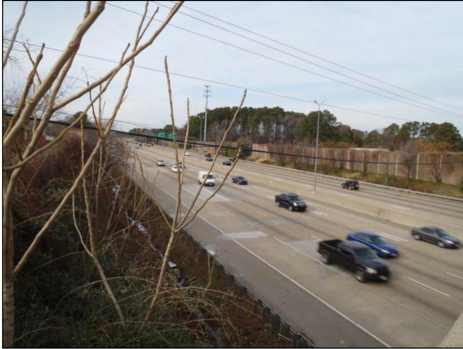
Photo 7: View along Eastbound Lane of I-64 Showing the Drainage Ditches and Sound Barriers in the Study Area.
