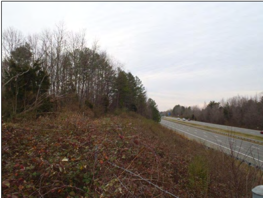
Photo 8: View East from the Stony Run Parkway Overpass along the Ridge above a Steep, Graded Slope Down to I-64.
