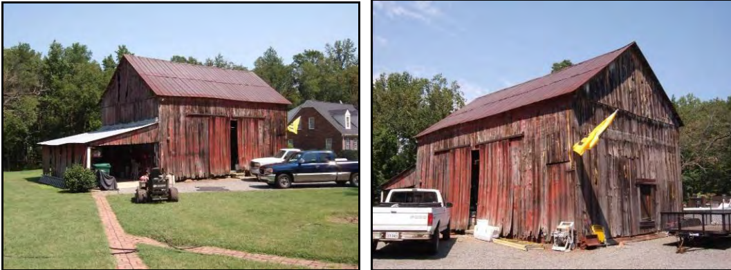
Photo [GROUP] 13: Southwest Oblique [LEFT] and Southeast Oblique [RIGHT] Views of Wood-frame Barn (Dovetail, Sep. 2011).
