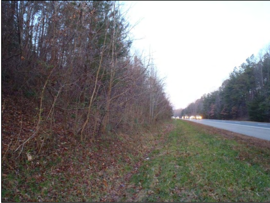
Photo 1: View West along the Eastbound Side of I-64 showing the graded slope and ditch near mile 230.
