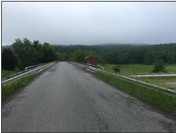
Picture 5: Route 690 Overpass
