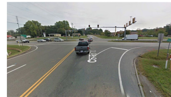
Route 29 and Route 703, Chatham, VA
