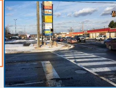
Southbound Approach (Route 1)
