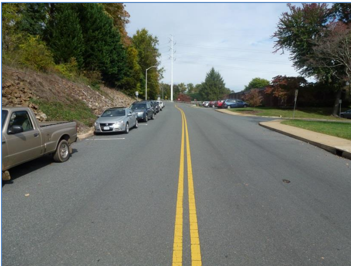
Figure 2. Gentry Lane, looking north. Wide travel lanes on Gentry Lane allow motorists to drive at speeds perceived faster than posted speed limits.
