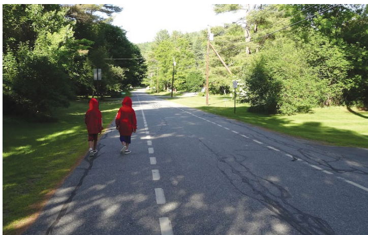
Figure 22. Example of an advisory shoulder in Hanover, New Hampshire. Photo from Western Transportation Institute.
