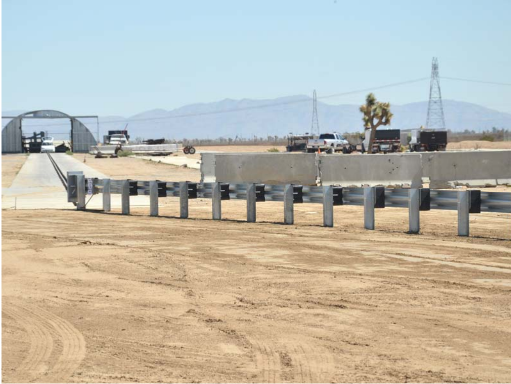
FIGURE 29. Pre-Test Left Rear \frac{3}{4} View of Test Article
