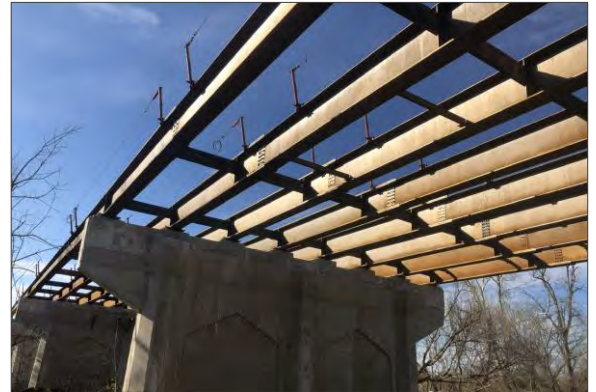
Figure 5.4: Chatham Bridge Pier Cap Extension
