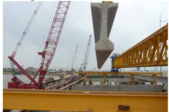
Figure 5.9: Galveston Causeway Bridge Girder Erection from Trestle with Beam Launcher
