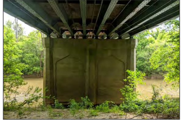
Figure 5.4: Chatham Bridge Pier Cap Extension
