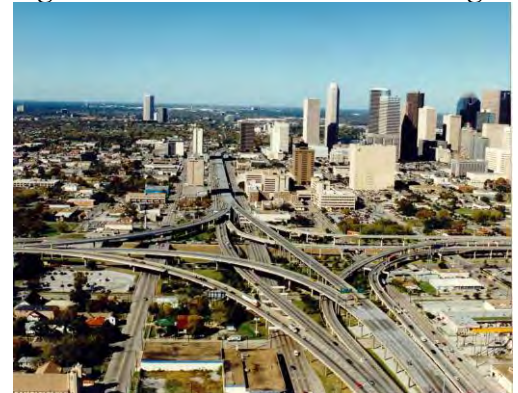
Figure 4.4: IH-45 Pierce Elevated Bridge
