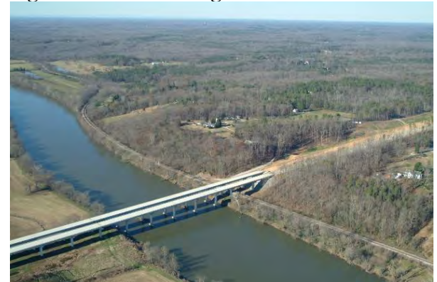
Figure 4.2: Rte 288 Bridge over James River PPTA
