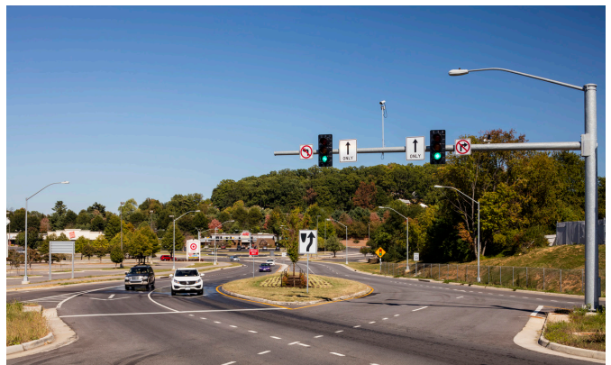
The I-581/Valley View Interchange was not originally envisioned as a DDI—this came about through the D-B process.
