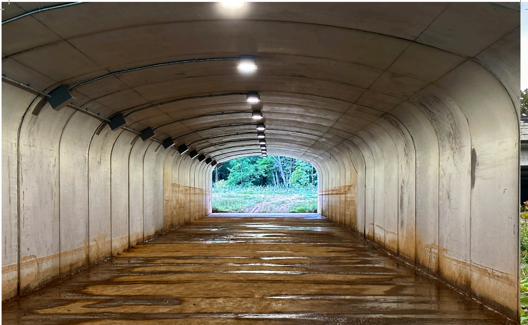
Above: Under Construction— Route 7 Corridor Improvements. Pedestrian underpass.
