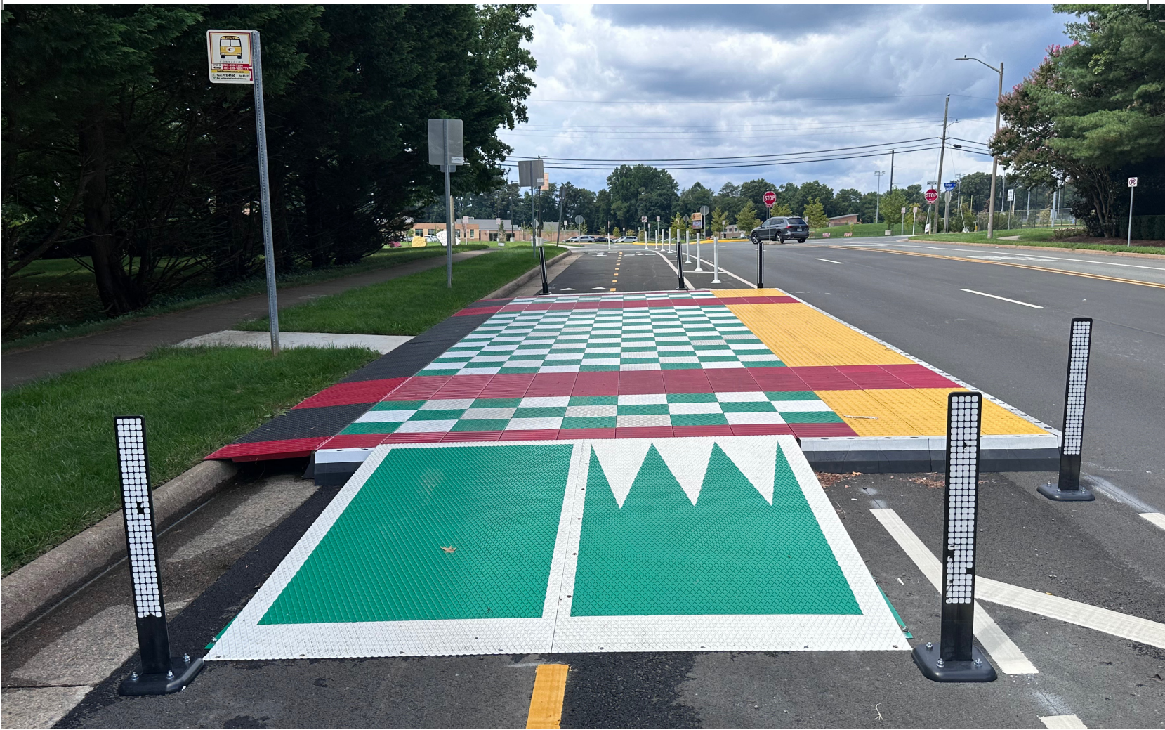
Above: "Zicla" modular bus platform in the cycle track on Country Creek Road in Fairfax County which provides pedestrians a boarding platform to buses in the vehicular travel lane.
