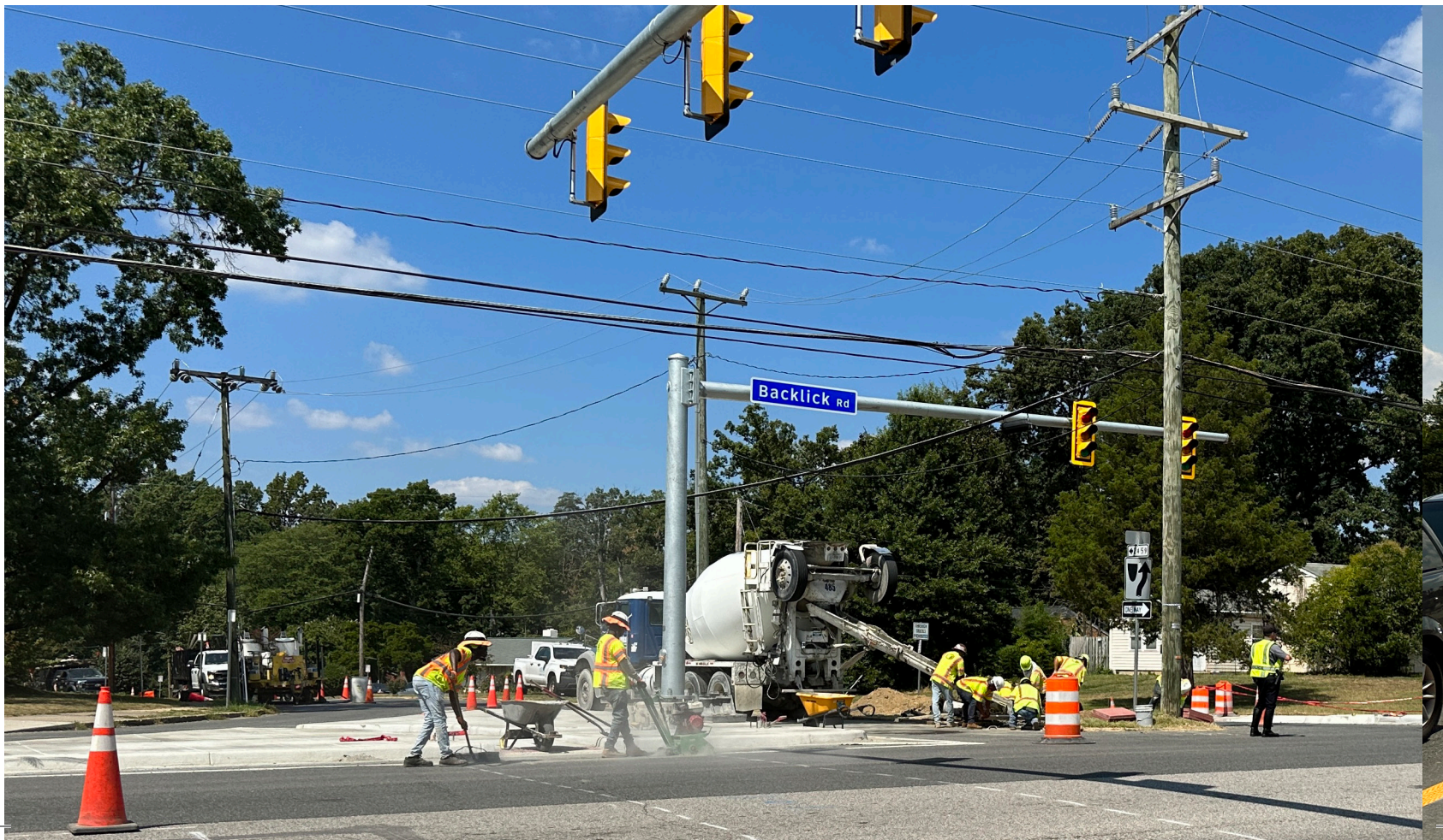
Below: Under Construction — Backlick Road and Leesville Boulevard Intersection Improvements
