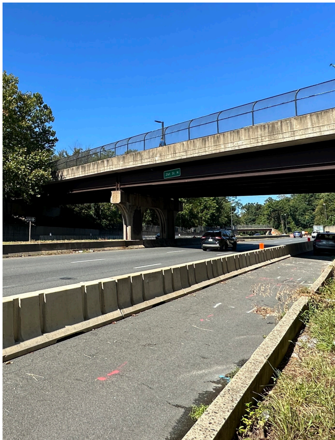
Above: Under Construction — 21st Street North over I-66 Bridge Rehabilitation
