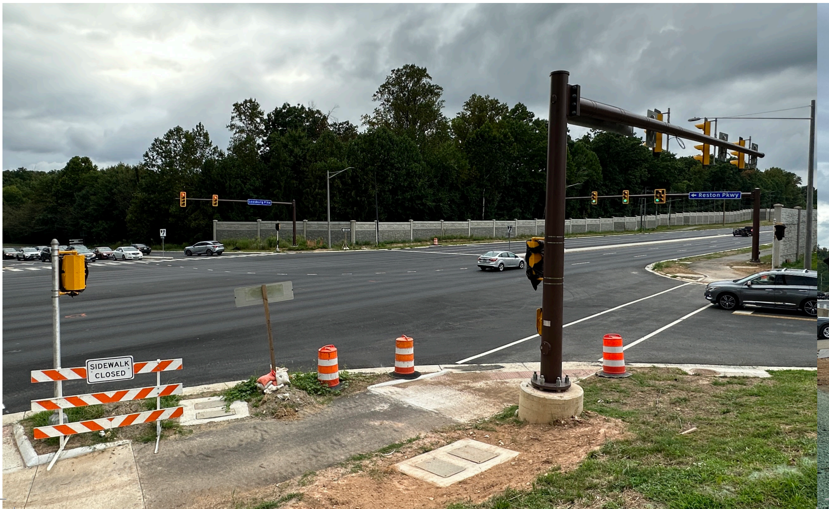
Below: Under Construction— Route 7 Corridor Improvements. Leesburg Pike at Reston Parkway.
