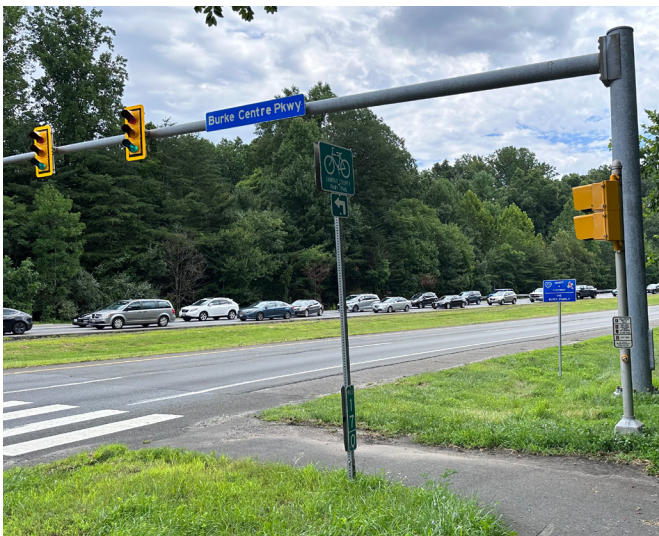
From top: In Design — Fairfax County Parkway Widening at Burke Center Parkway.
