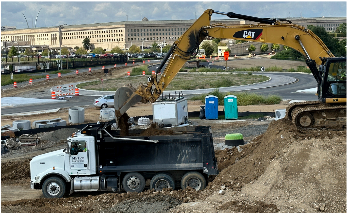
Above: Under Construction — Boundary Channel Drive at I-395 Interchange Improvements
