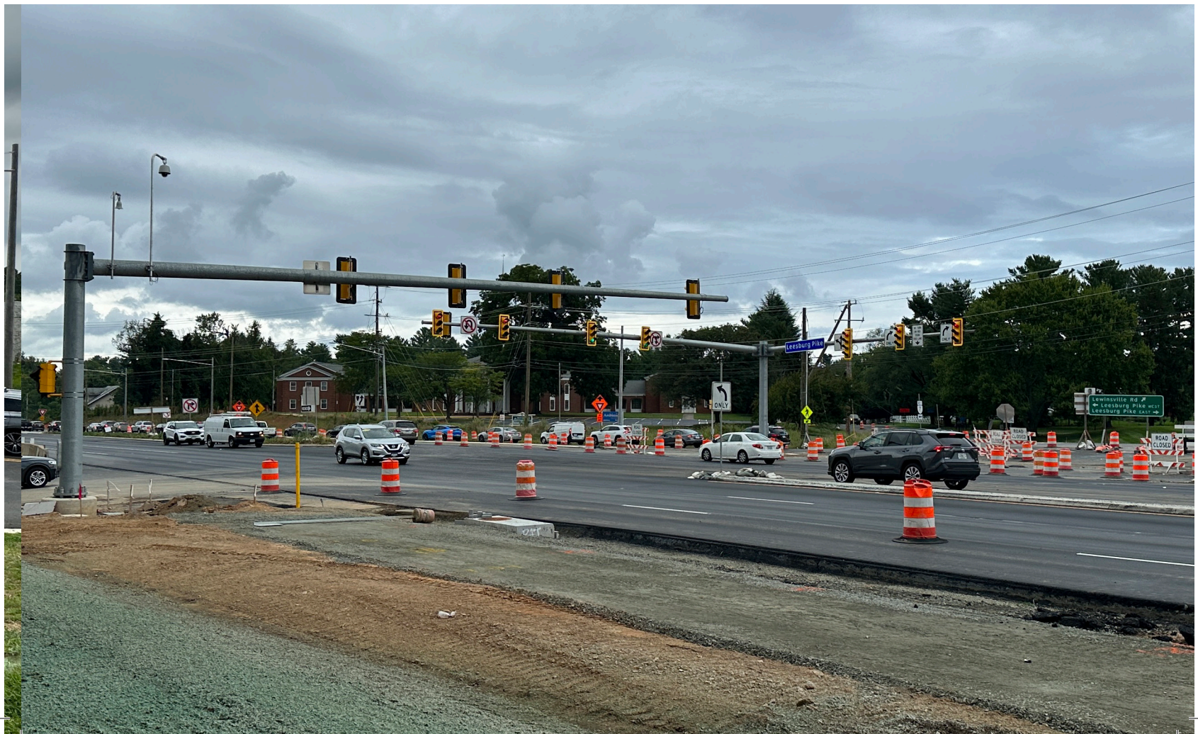
Below: Under Construction— Route 7 Corridor Improvements. Leesburg Pike at Lewinsville Road.
