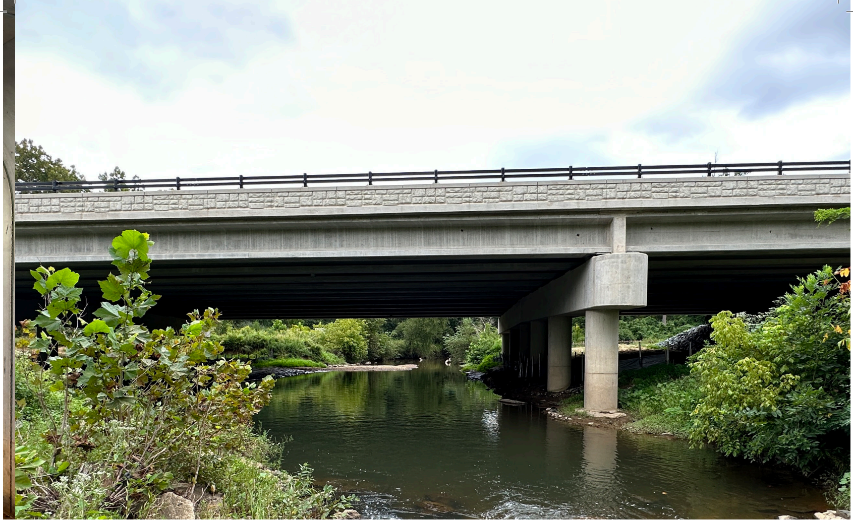
Above: Under Construction— Route 7 Corridor Improvements. Bridge over Difficult Run.
