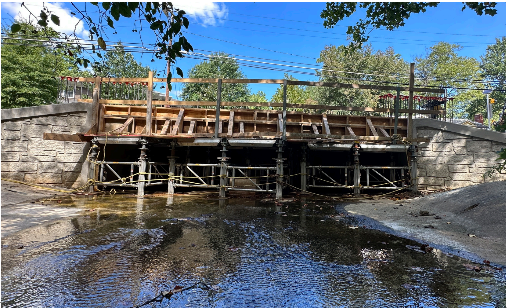
Below: Under Construction — South Oak Street over Tripps Run Bridge Replacement
